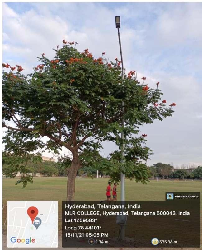
LED Lights in ground at MLRIT
